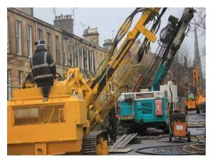
Drilling work was carried out from the streets surrounding the blocks using versatile Casagrande C6 rotary percussive drilling rigs with multi-angling kinematics and smaller Halco 450 rigs which were used in the more restricted back gardens areas.
