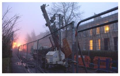
This scheme was carried out for Glasgow City Council and involved treatment of shallow coal workings beneath 3 large residential housing terraces in the Strathbungo Conservation Area. The scheme was secured on a combined Quality/Price tender submission with specific emphasis on proposed methods of work, programme, public relations and management of environmental risks.
